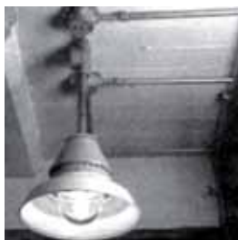
Typical Class 1 Div 1 conduit installation
