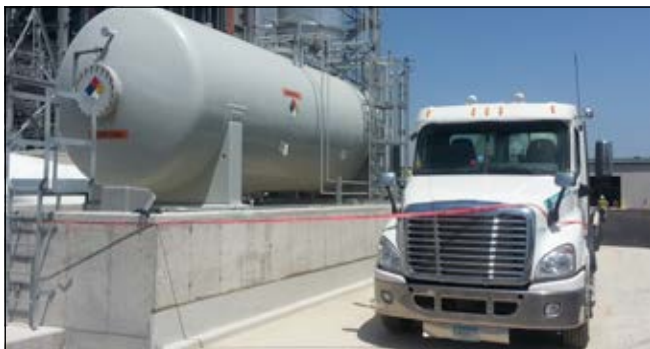
High-visibility magnetic level indicator with magnetostrictive transmitter supports the offloading of ammonia at a combined cycle power plant
