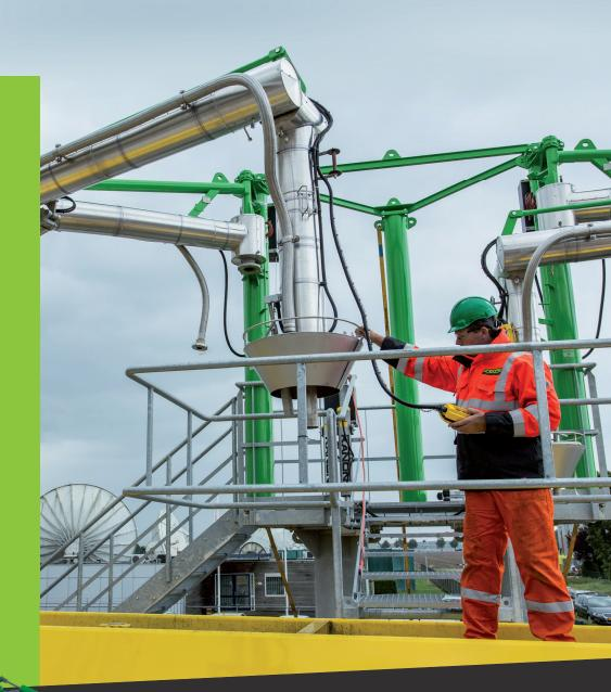
KANON loading arms are suitable for transferring virtually all kinds of liquids and gases, regardless of whether they are toxic, corrosive or having extreme temperatures.
