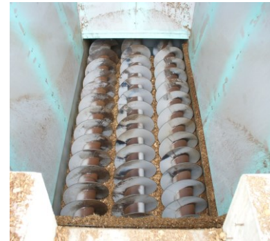
Mounting in discharge screw (wood-fired power plant)
